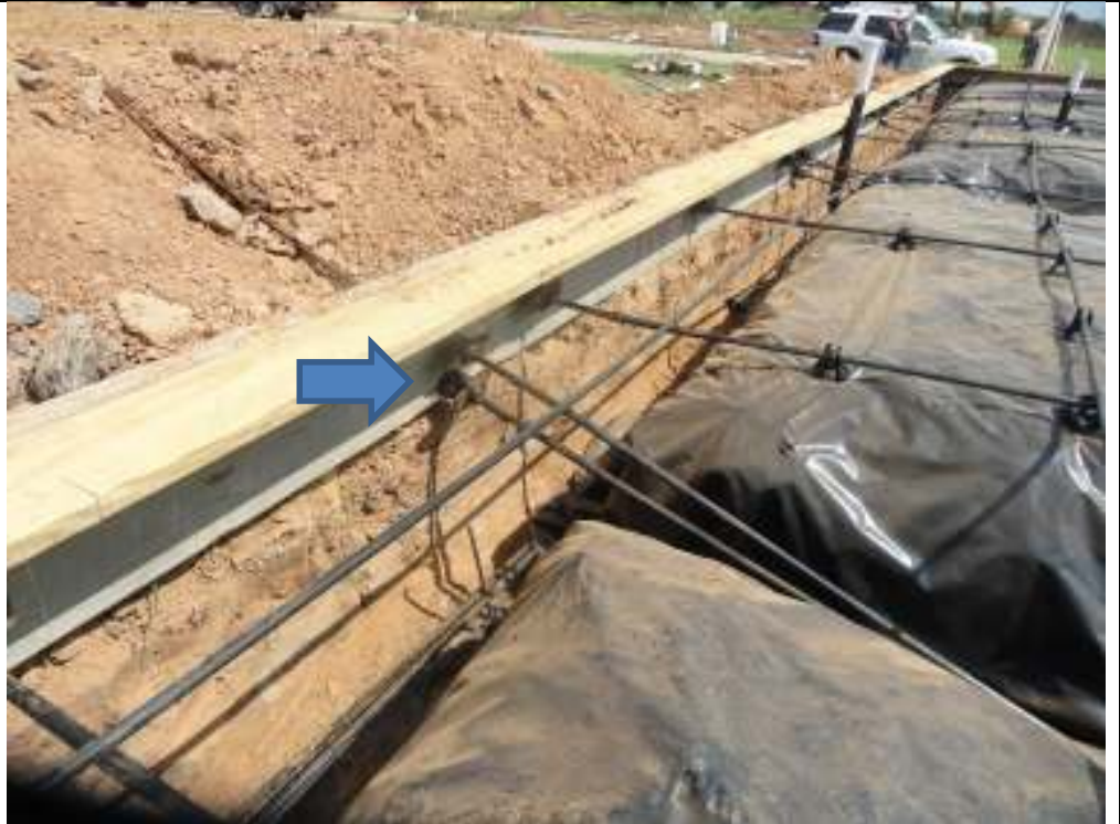
PHOTO 13 POCKET FORMER MUST BE FLUSH WITH FORM BOARD
