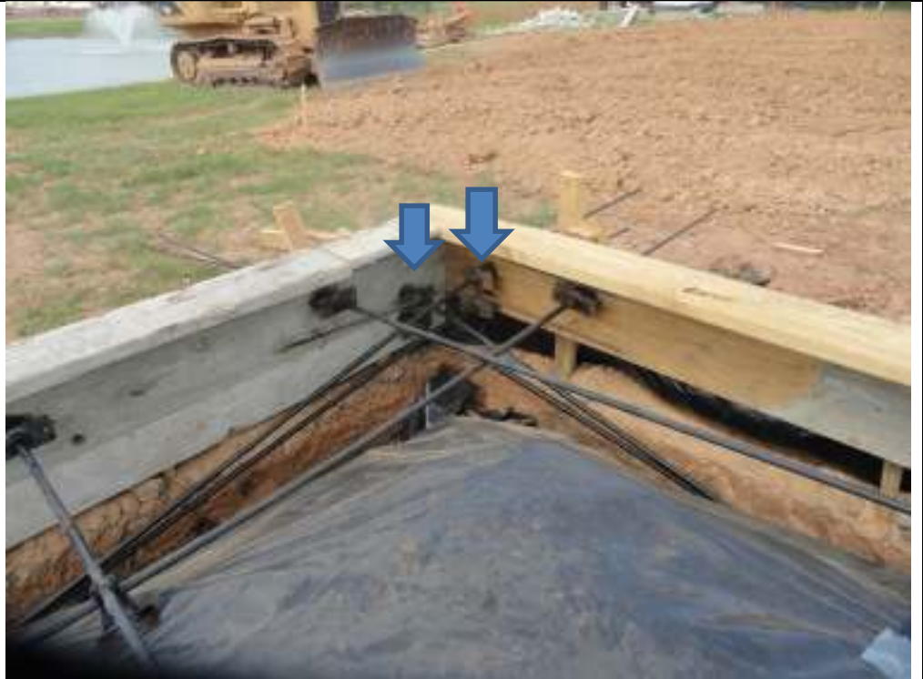
PHOTO 11 MASTER BEDROOM ANCHOR NAILERS MUST BE AT LEAST 6" FROM THE CORNER
