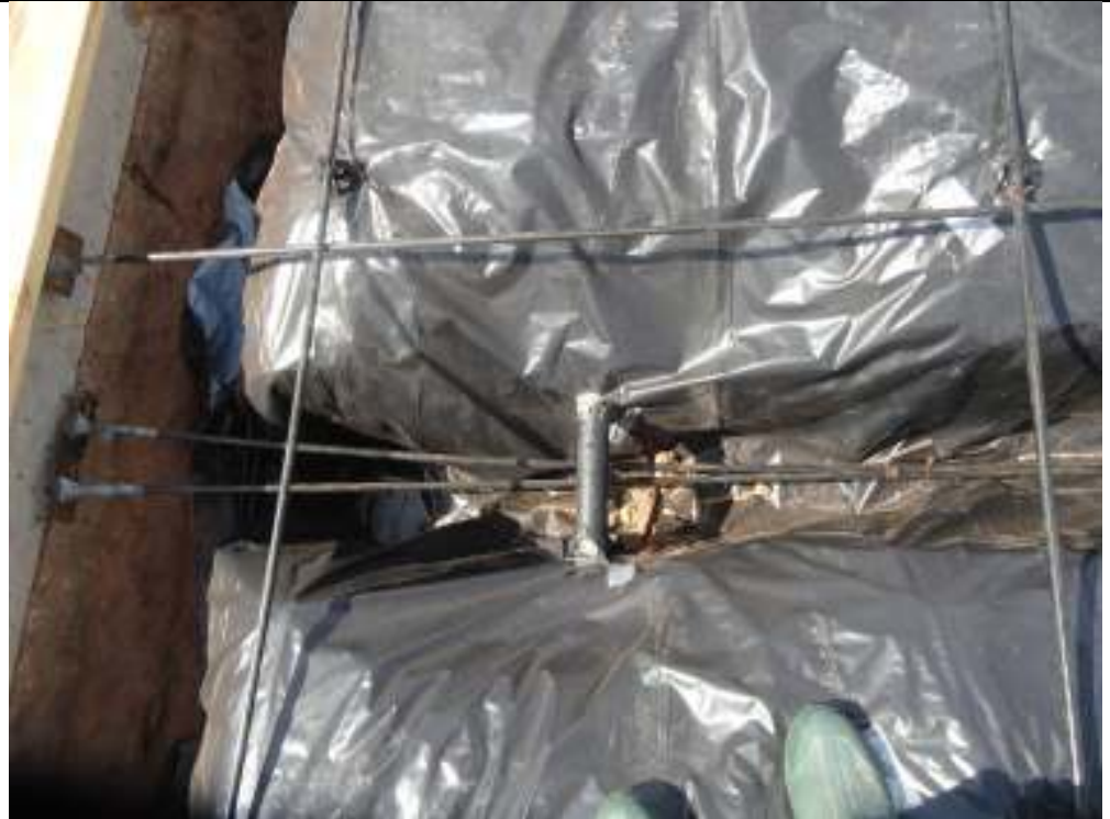
PHOTO 3 TAPE UP POLY WRAP TEARS UNDER PIPE NEAR WINE RACK REMOVE TRASH
