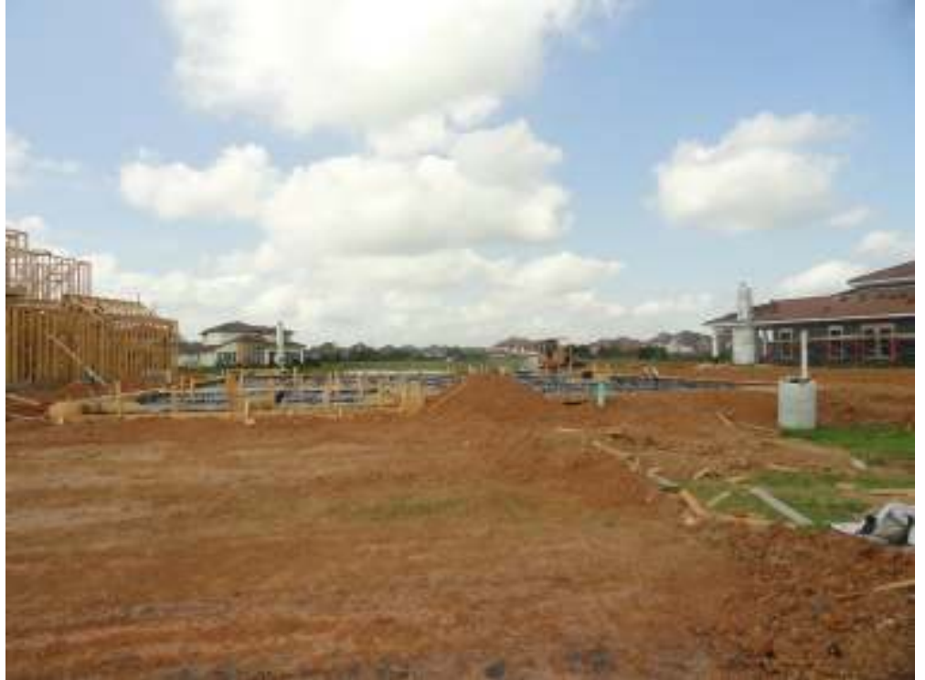
PHOTO 1 3903 SUNDANCE HILL FRONT ELEVATION AT PRE FOUNDATION STAGE
