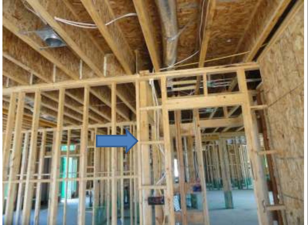
PHOTO 19 COMPLETE FOAM SEALANT AT STORAGE ROOM ADJOINING GARAGE
