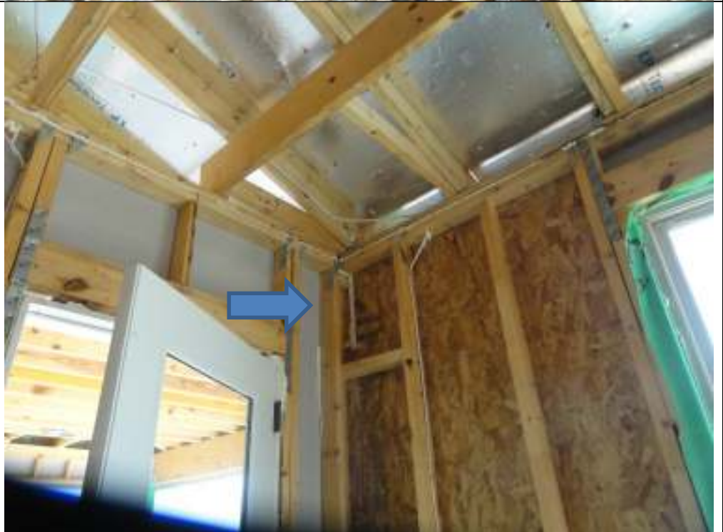
PHOTO 14 EXTEND VAPOR BARRIER TO TOP OF GUEST BEDROOM WALL
