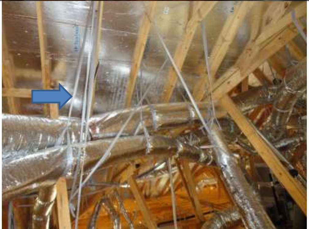
PHOTO 24 EXTEND PURLIN 4 RAFTERS AND ADD TWO SUPPORTS. RAFTERS LOAD NEEDS TRANSFERRING (OVER ATTIC LADDER).
