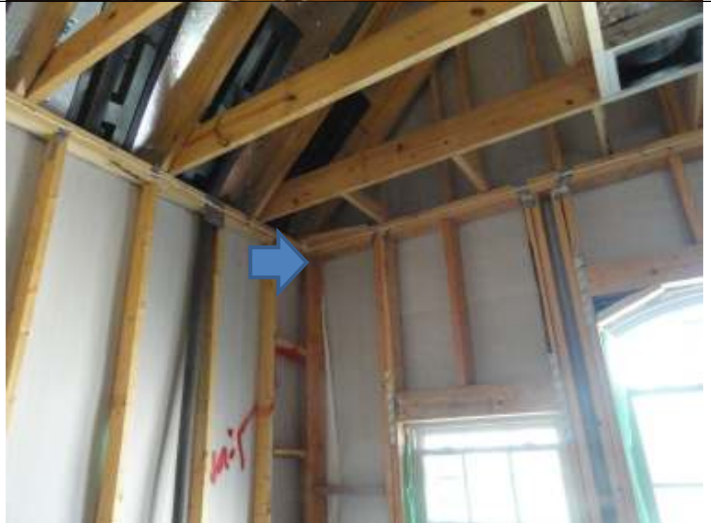
PHOTO 22 EXTEND VAPOR BARRIER OVER TOP PLATE AT FRONT CENTER BEDROOM CORNER
